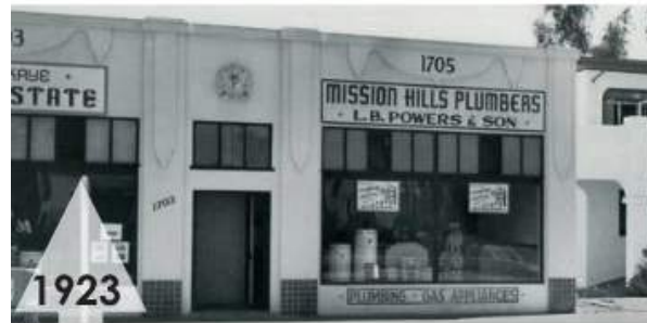
Mission Hills Plumbers 1923
