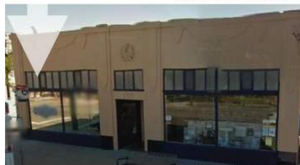
Mission Hills Plumbers
